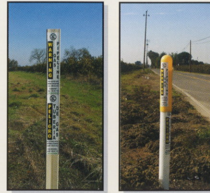
A pipeline marker similar to one of the markers pictured above will be used to show the approximate location of Lodi Gas Storage's pipeline.
